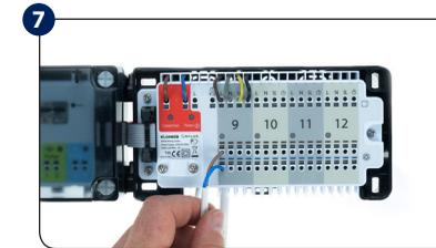
Connect the thermoelectric actuators wires.
